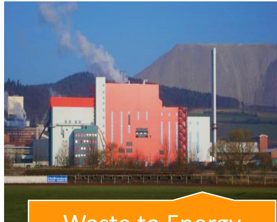
Waste to Energy Projects
