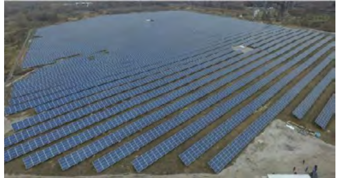
Solar Power Plant as seen from the drone (CNW Group/TIU Canada)
